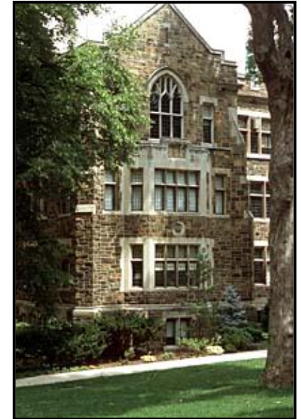
Packard Laboratory, Lehigh University Department of Mechanical Engineering & Mechanics
